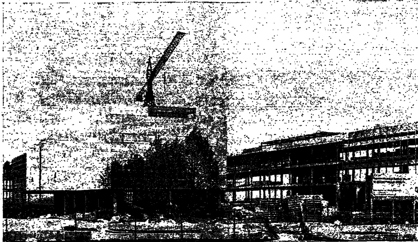
Construction of the shopping centre has greatly buoyed commercial confidence in Milton Keynes. Here Ashton House and Norfolk House, two office blocks, are under construction in the city centre
